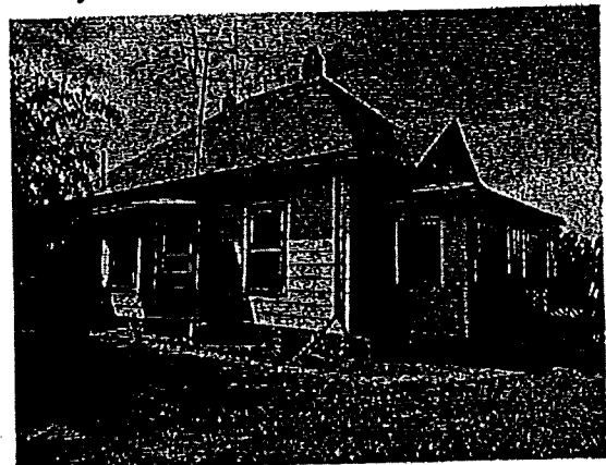
Dickey House Exterior - Southeast Side
