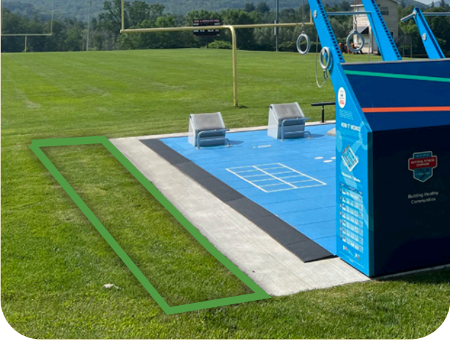
Acceptable typical edge conditions include grass, artificial turf, landscape planting, mulch, hardscape or other rubber surfacing material.
