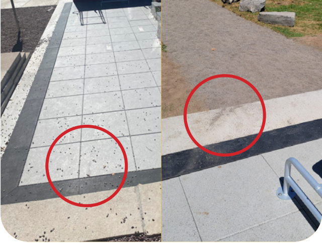
Unacceptable edge conditions include gravel, sand, decomposed granite, and other loose material. These materials cause tripping hazards and maintenance issues
