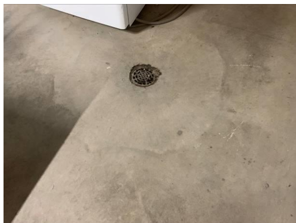
10. View of interior floor drain located within the Pride Mechanical warehouse
