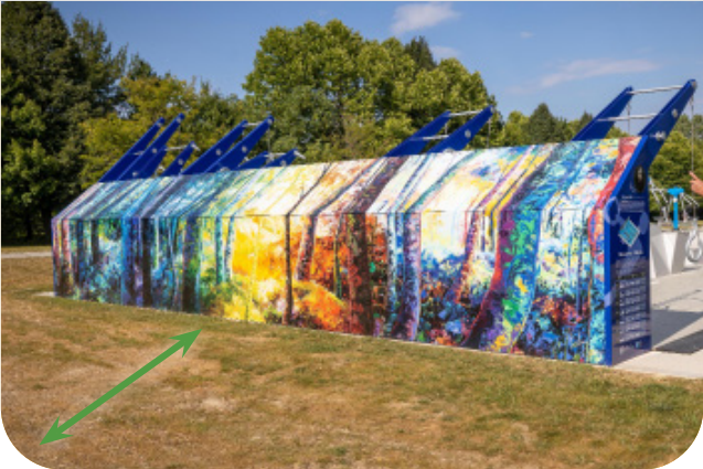
Fitness Courts® are required to be placed at least 25’ away from all vertical structures including but not limited to brick walls, fencing, retaining walls. The Fitness Court® Wall orientation should be perpendicular to the connecting pathway and vertical surface allowing clean safety sightlines.
