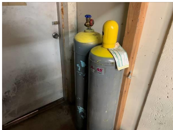
12. View of compressed gas cannisters located within the Pride Mechanical warehouse
